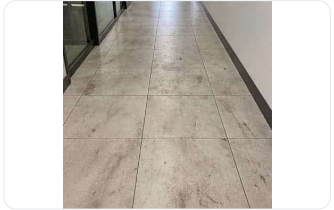
Aged floor tiles marked for detailed floor cleaning 06:13 pm
