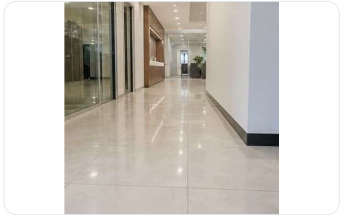
Office hallway floor clean, dry, and ready for trade
